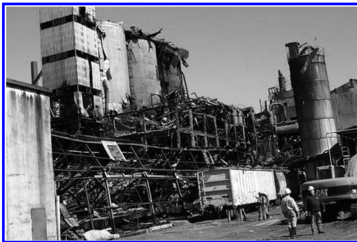
Figure 28. Aftermath of Port Wentworth Georgia sugar refinery explosion
