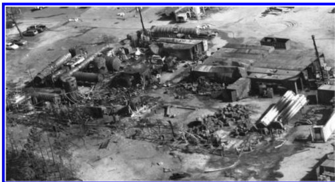
Figure 8. Aerial photograph of T2 site taken December 20, 2007 after reactor explosion. Photograph courtesy of U.S. Chemical Safety and Hazard Investigation Board, taken from Investigation Report No. 2008-3-I-FL, September 2009
